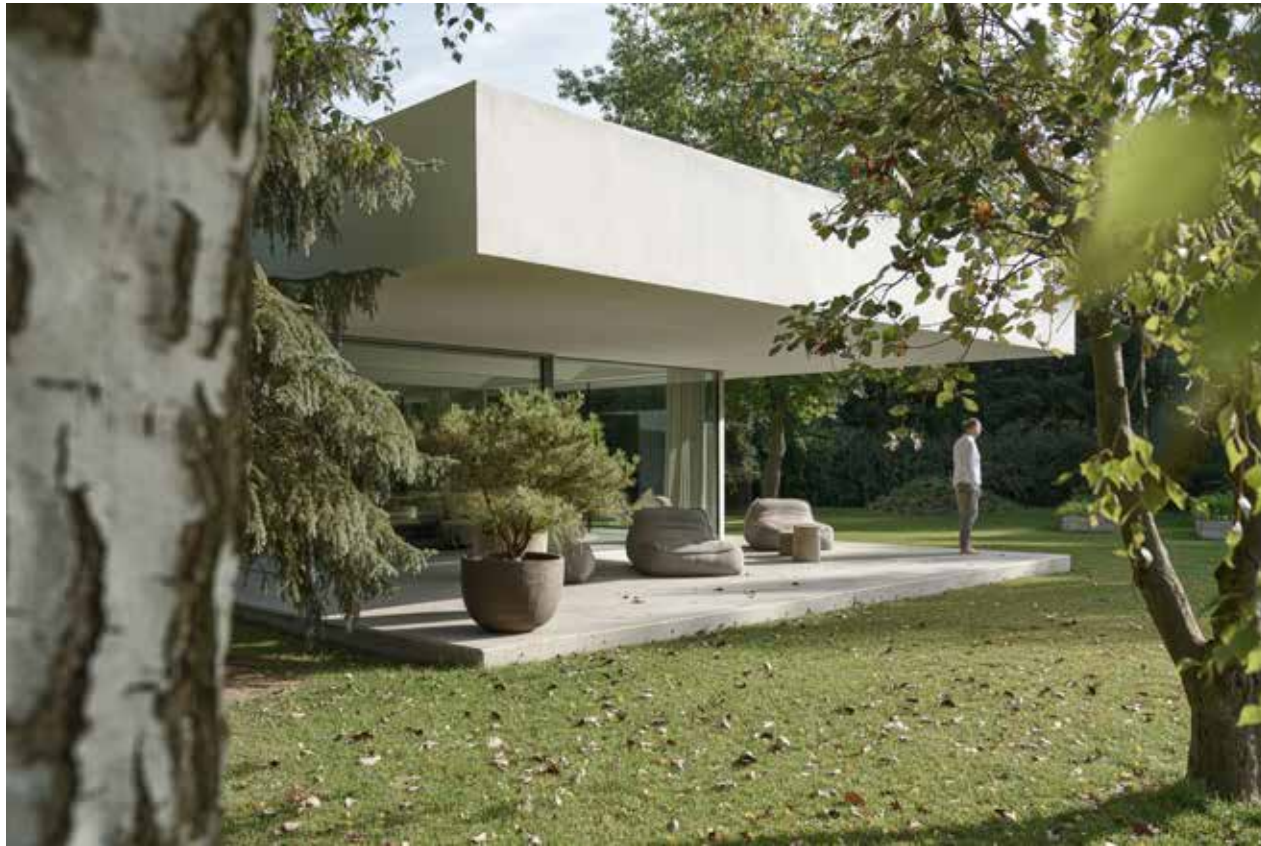
The architectural studio PL Architekci based in Poznan chose to use AU and U vessels for the terraces.
